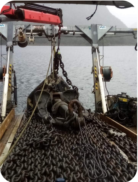
Removing damaging old anchor and chain moorings
